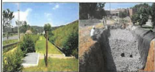
침투도랑(Infiltration trench)
